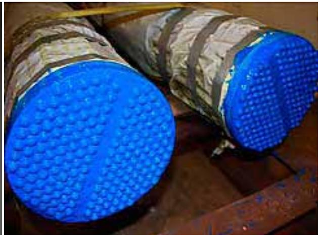
**Coating in progress, epoxy coating encapsulates surface in a protective film; tube end plugs protect from over coating down tube.**
